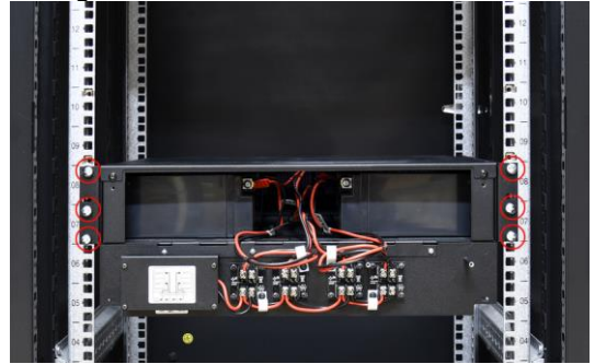
Fig. 4 The battery mounting method.
